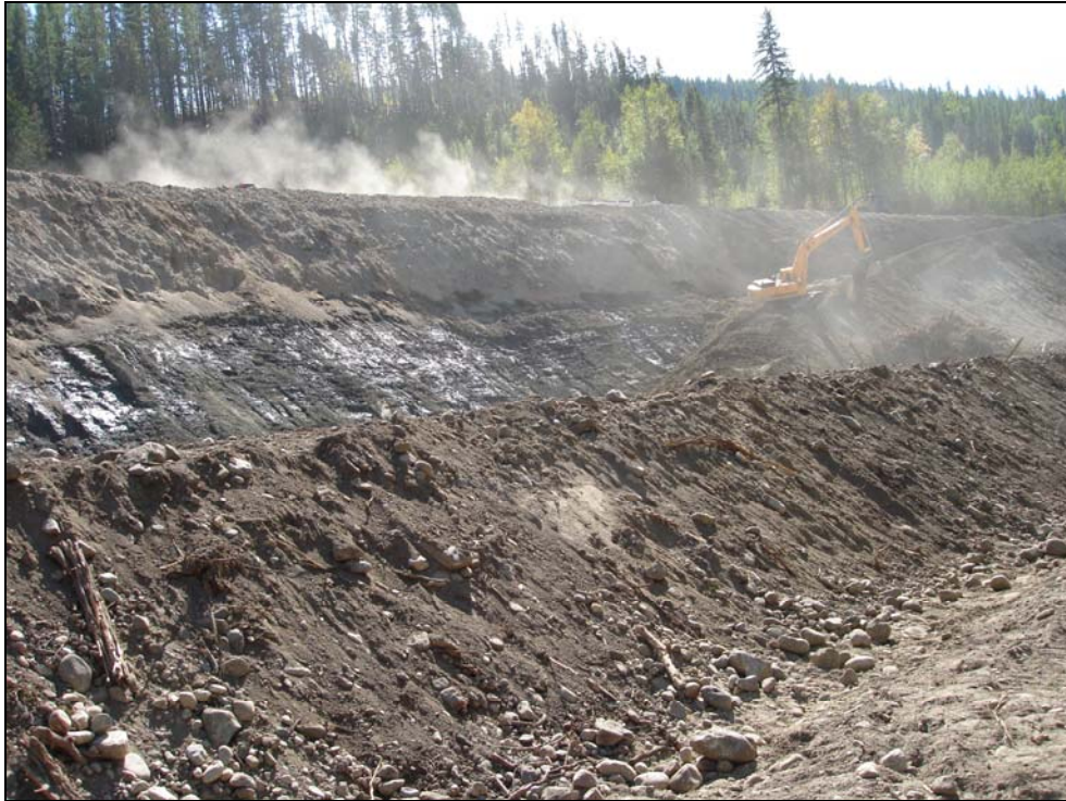
Extraction excavation south of Mission Creek
