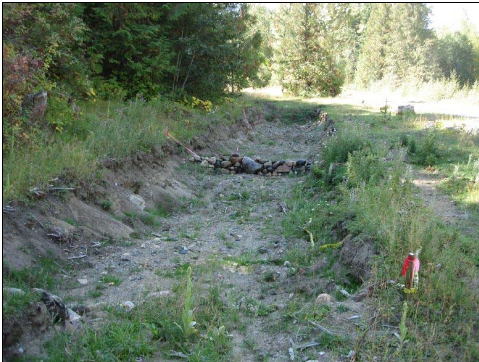
25 cubic metre drainage sediment control pond volume for a 10 acre site
